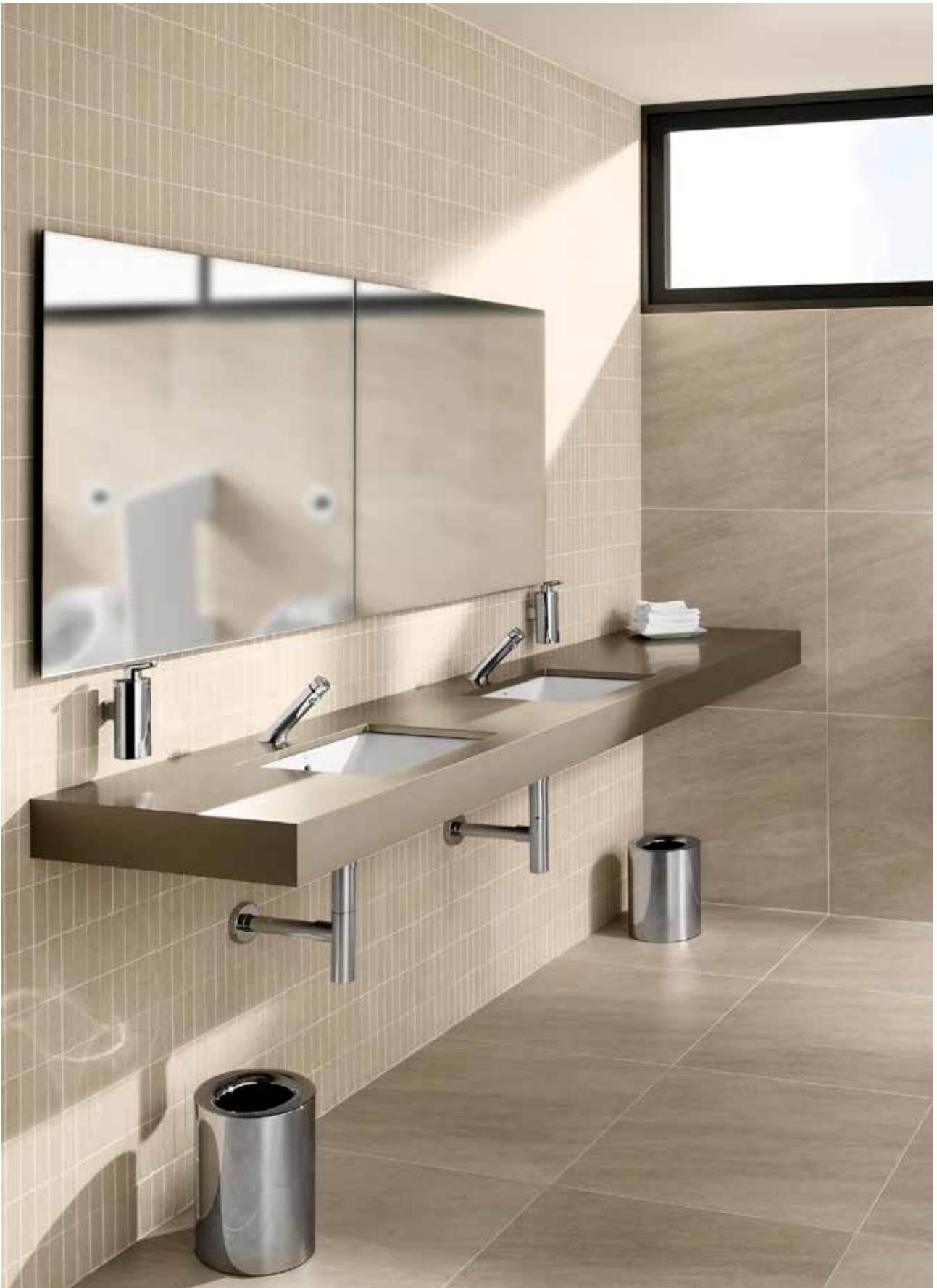
Diverta wash basin countertop, Avant faucet and Hotel's accessories.
